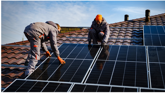
The Case for Sustainable Roofs
