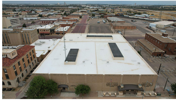
Lubbock County Law Enforcement Center Benefits from Roofing Project
