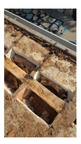
The repair for this roof required extensive framing and sheathing replacement and a new roof system above the plywood diaphragm that included a vapor retarder, 2 staggered layers of 2" polyisocyanurate insulation, a tapered polyisocyanurate insulation to provide a 1/4" per ft slope, ½" high density polyisocyanurate cover board, and mechanically fastened thermoplastic single ply
