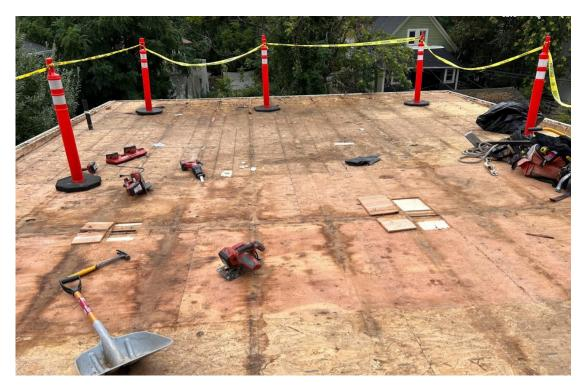
Within five years, the underlying OSB sheathing had deteriorated. Apparently, the closed cell spray foam insulation either did not bond to the adjacent rafters and/or was not installed continuously
