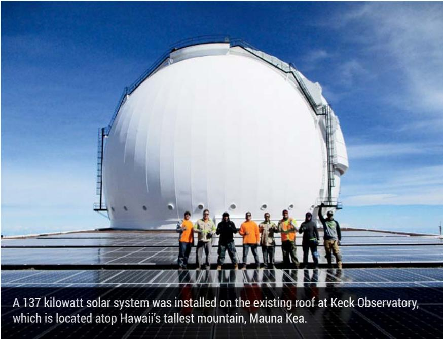
A 137 kilowatt solar system was installed on the existing roof at Keck Observatory, which is located atop Hawaii's tallest mountain, Mauna Kea.
