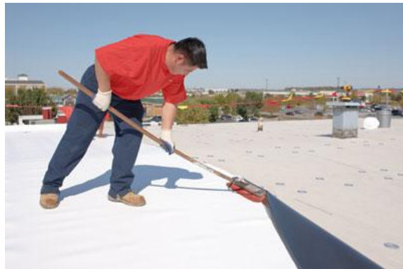
A Firestone worker installs UltraPly TPO roofing membrane.
