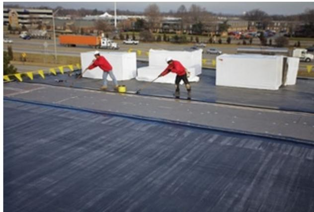
Workers install a Firestone RubberGard R.M.A. System, an EPDM roof. Firestone, like most of its fellow members of the EPDM Roofing Association, makes both EPDM and TPO roof membranes.
