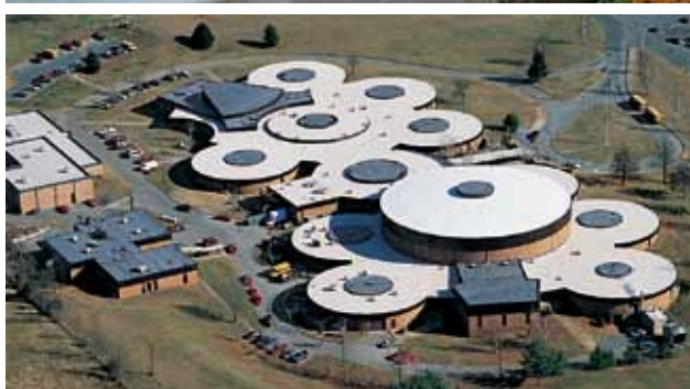
The development of complementary technologies has allowed EPDM to be beneficial in a wide number of applications, including plaza decks and larger projects using white EPDM membrane. Pictured (above) is a plaza deck paver system installed over a 145-mil EPDM system and (below) a white EPDM roof system.
