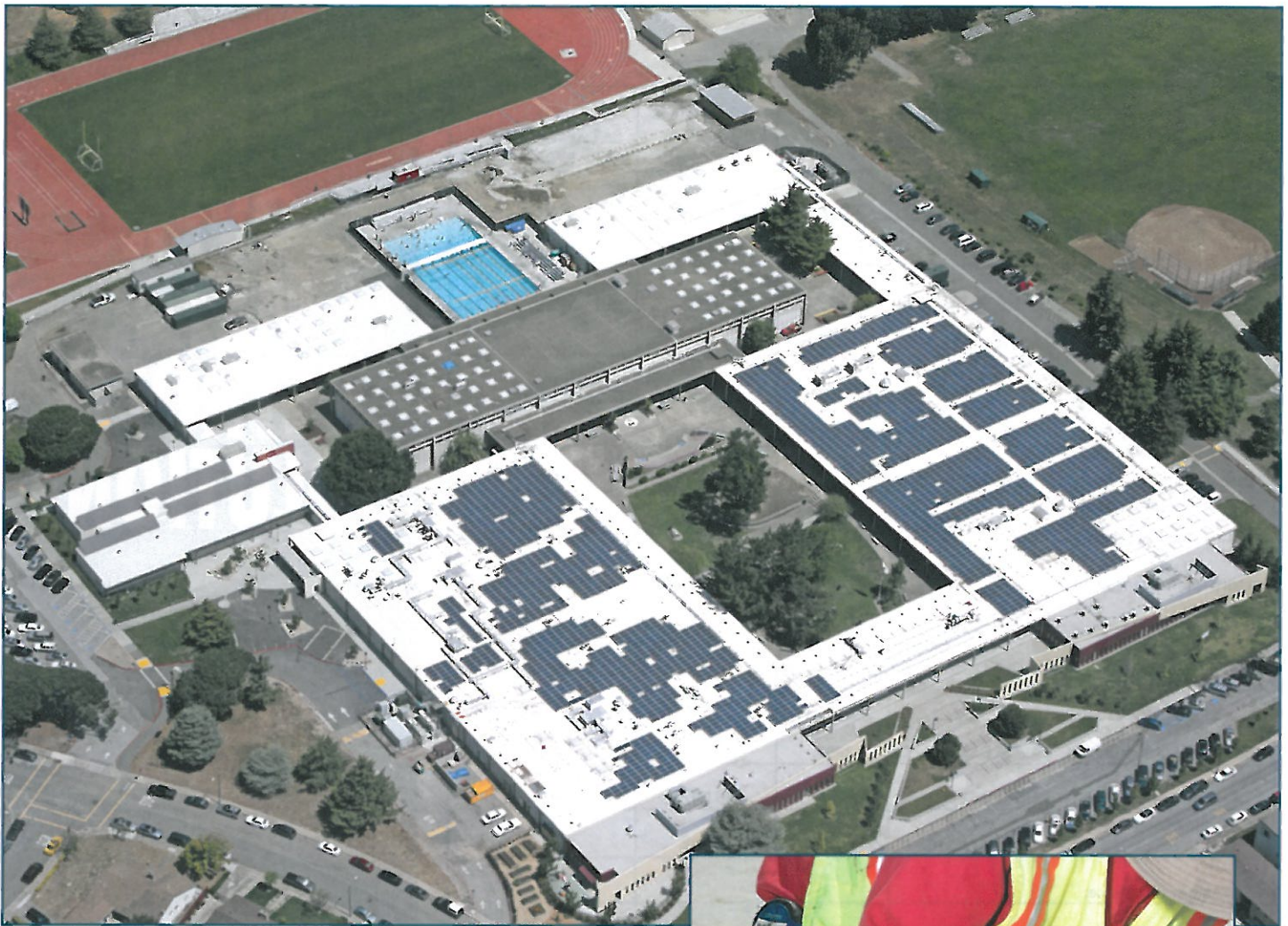
Photo 1 – White EPDM roofing membrane serves as a high-performance foundation on a multifacility reroof project for the San Mateo Union High School District that featured more than 2,500 photovoltaic panels installed atop three California high schools.
