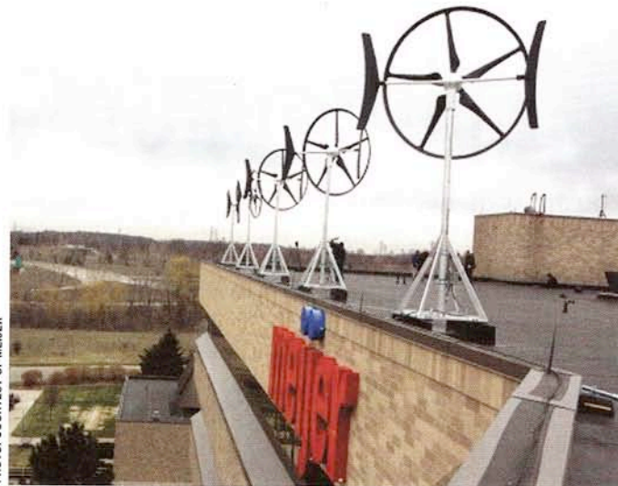
This retailer installed wind turbines on its roof. Equipment like this that rises above the roof surface significantly needs to be accommodated to ensure it stays in place.
