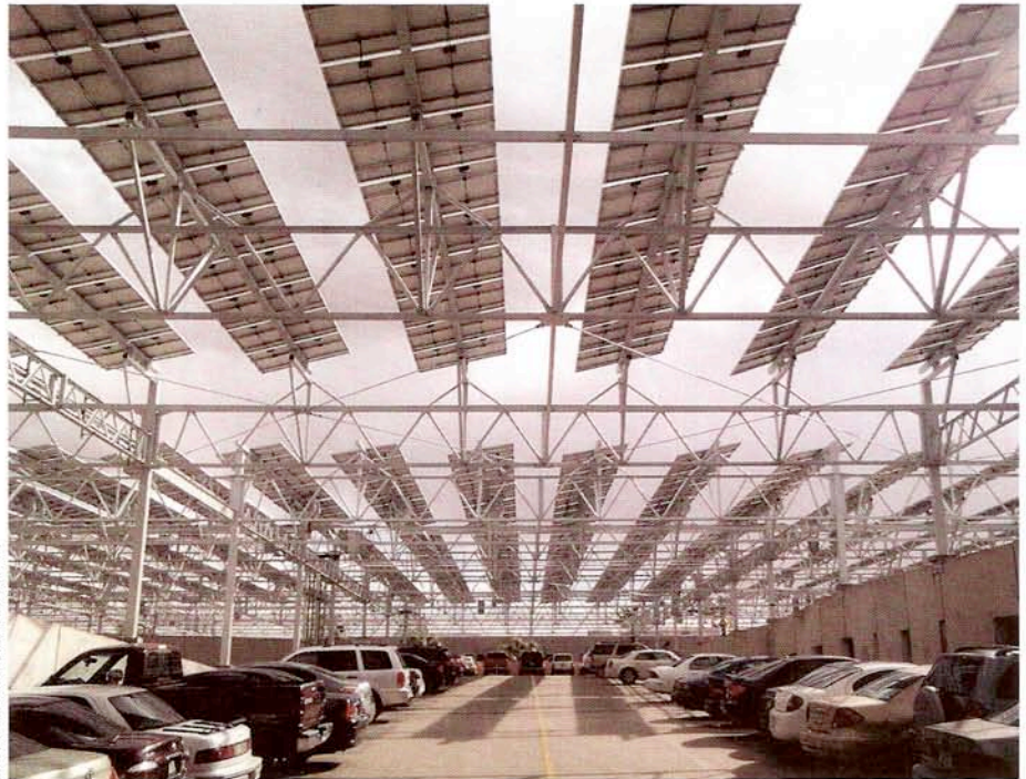
Solar panel systems are sometimes sited above open spaces. In this case, the structures that surround the parking lot play a part in supporting this installation.
