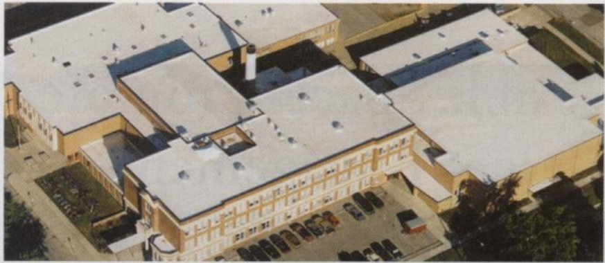
Photo courtesy of CertainTeed Commercial Roofing
