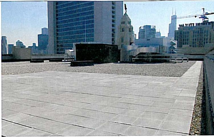
Concrete pavers and gravel ballast meet Chicago Energy Conservation Code requirements and do not require any care or cleaning to maintain.
