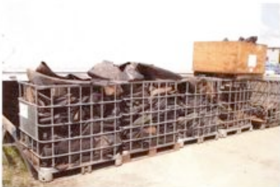
■ Recycling baskets from WDG allow roofing contractors to quickly package EPDM membrane for transport.
