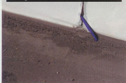
Photo 1: The soiling of this white membrane has resulted in a surface color darker than what would be experienced on a smooth-surfaced black roof covering. Photos courtesy of Hutchinson Design Group Ltd., Barrington, Ill.
