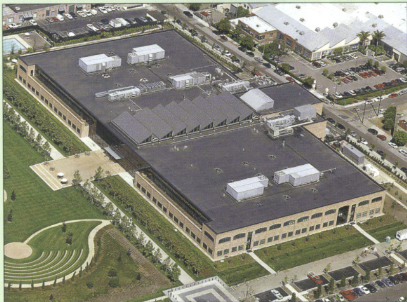
At the Pixar Animation Studios building in Emeryville, California, a 10,229-m 2 (110,100-sf) fully adhered ethylene-propylene-diene-monomer (EPDM) roofing membrane helps protect the people—and computers—that brought forth Toy Story, The Incredibles, and Finding Nemo.
